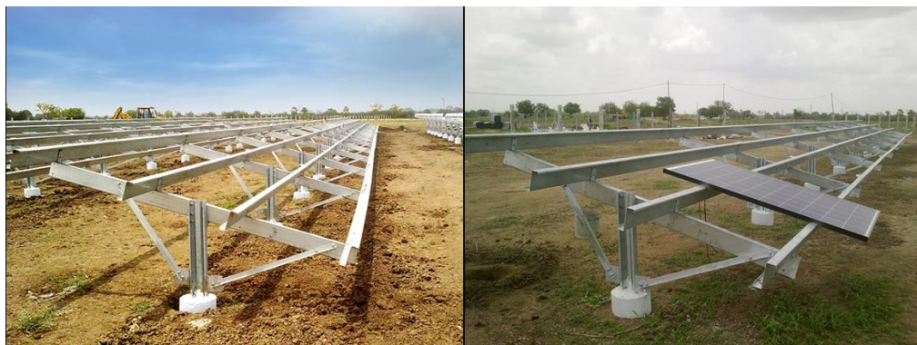
Figure 3-6 Solar power plant civil work preparation.
