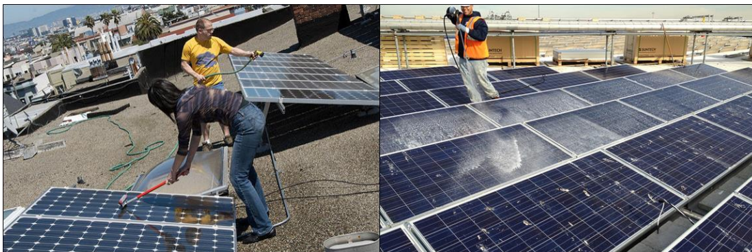
Figure 3-7 Mechanical system for supply water in solar power plant area.
