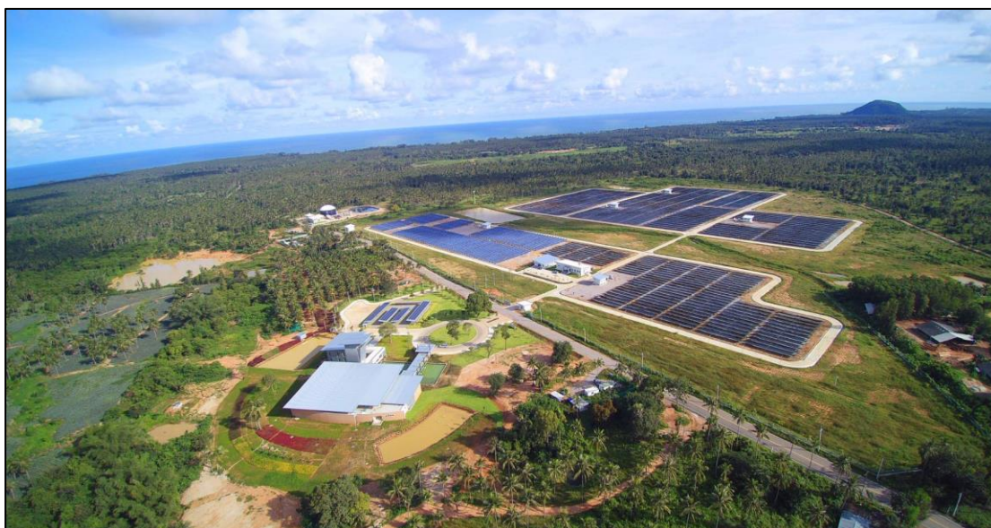
Figure 1-2 EGAT Thap Sakae Solar Power Plant, Prachaup Khiri Khan Provincial Thailand.
